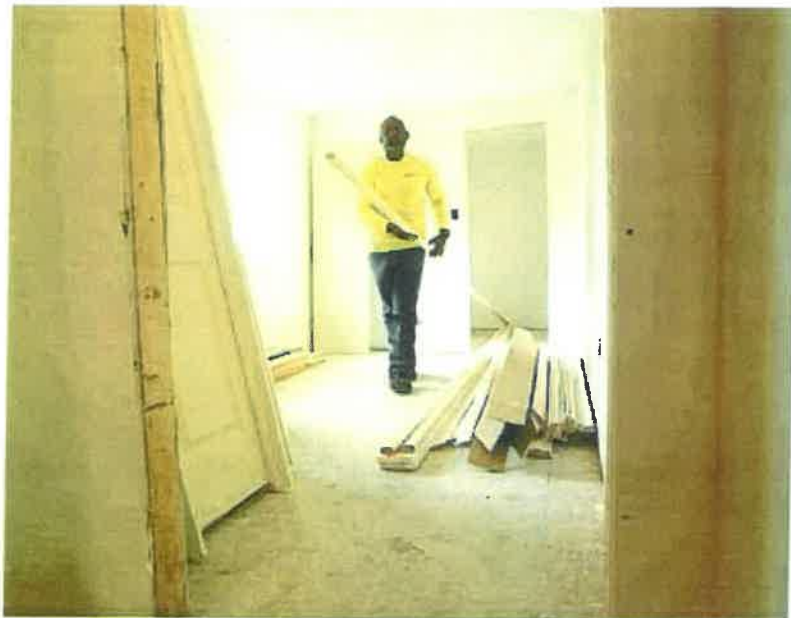
Olmos works inside the home on Tulpehocken Street.
